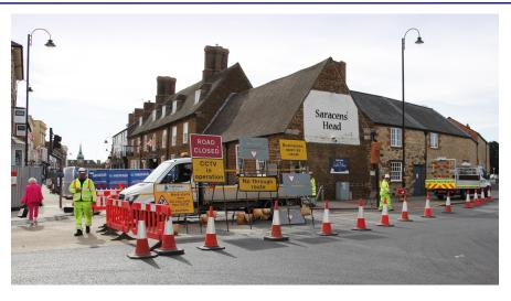
This was a high profile scheme involving essential maintenance work to 1.3km of the A5 Watling Street in Towcester, Northants to address various issues including poor highway drainage, extensive surface water ponding that was causing splash damage to properties and posing a significant risk to pedestrians, cracking and rutting of poor quality reinstatement to a 430 m long gas main trench installed in 2009 together with replacement of kerbs and footpaths damaged by vehicle encroachment.
